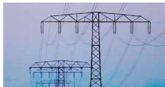
Electrical power pylons with high-voltage power lines are seen near Weselitz, Germany November 18, 2022. © Lisi Niesner/REUTERS
