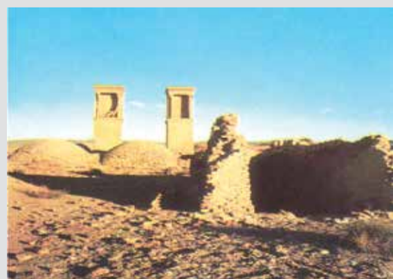
A large water storage tank with air traps near desert
