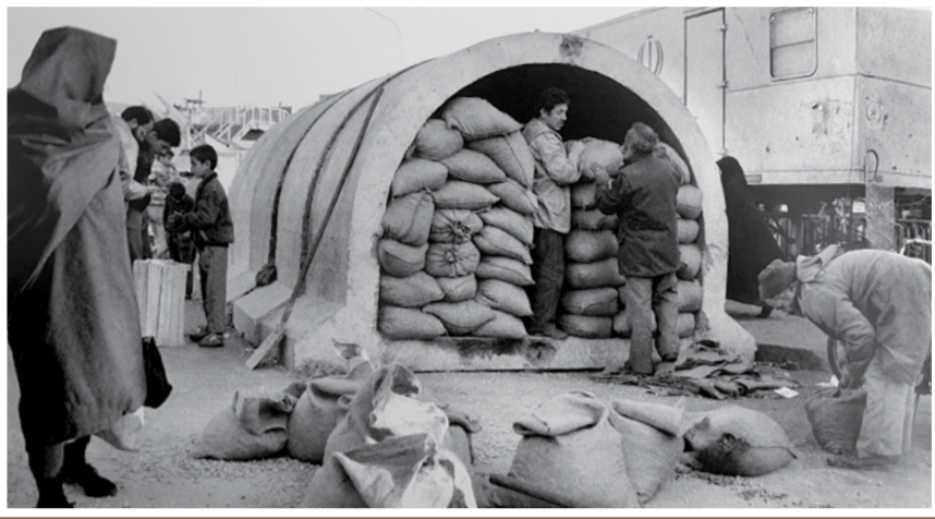
⤴ The construction and establishment of shelters on streets to protect people from Iraq's missile attacks in Tehran's Imam Hussein Square in March 1988
