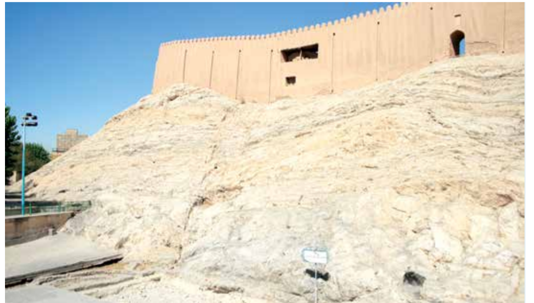
Cheshmeh Ali spring after drying up ● IRAN DAILY
