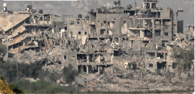
This picture shows buildings in the Gaza Strip that have been destroyed by Israeli bombardment on October 31, 2023. ● YURI CORTEZ/AFP
