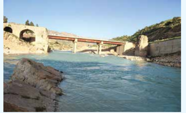
Qal'eh Dokhtar Bridge ● IRNA
