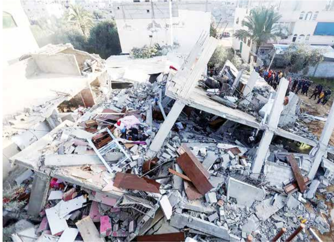
Palestinians inspect the site of an Israeli strike on a house, amid the ongoing war on Gaza, in Rafah in the southern Gaza Strip, December 17, 2023. REUTERS
