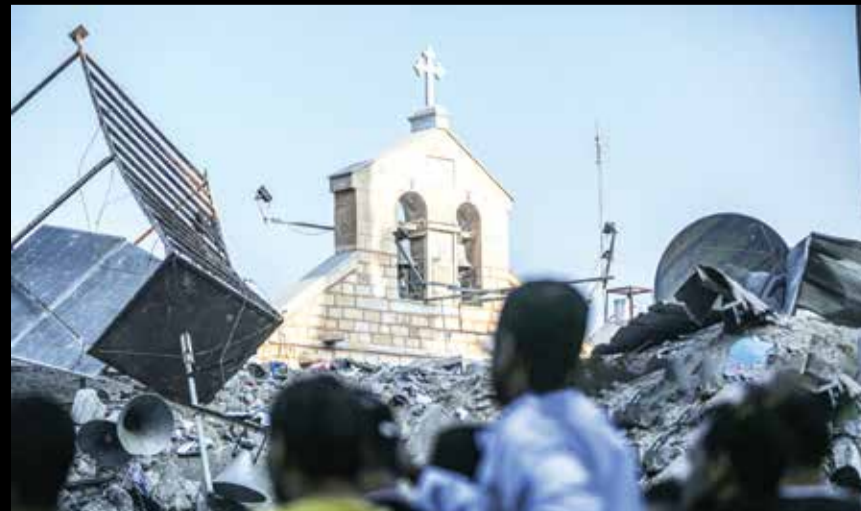
A view of the damaged historical Greek Orthodox Saint Porphyrius Church, where civilians took shelter, after an Israeli airstrike in Gaza City, Gaza, on October 20, 2023.
