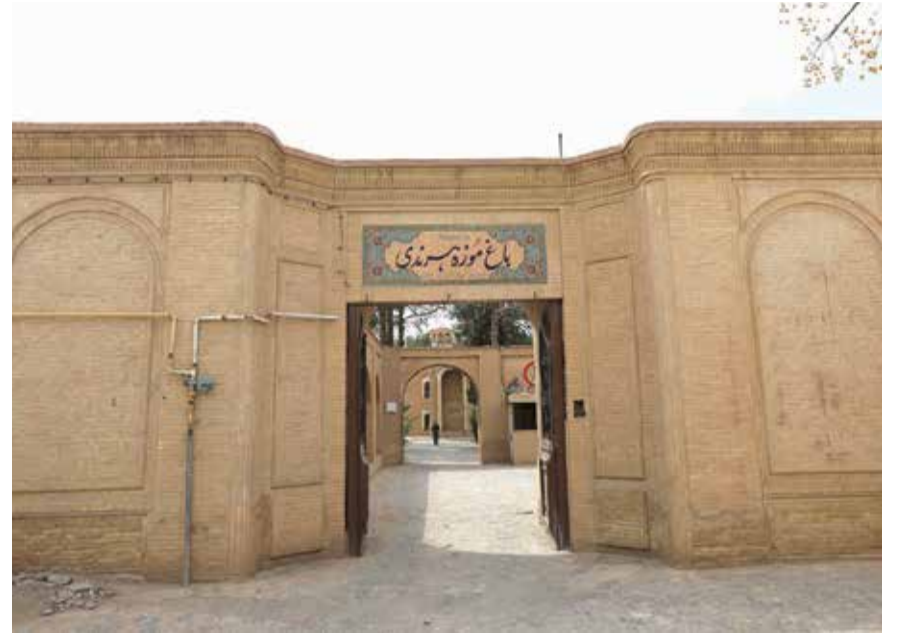
Central building ● chn.ir
