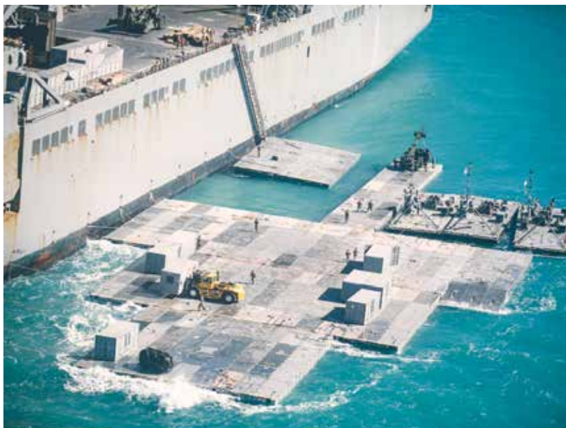
US Army personnel are seen on a floating pier off the coast of Bowen, Australia, last July. The US plans to construct a similar pier off Gaza. ● US ARMY PHOTO
