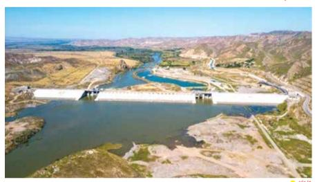
this species' conservation. Aras Dam boasts four Kaplan turbines, two on each side, each generating 11 megawatts, totaling 44 megawatts, revolving at 187.5 rounds per minute to yield a production capacity of 22 megawatts on Iran's side. The construction of this reservoir aims to bolster agricultural water supply in the region and facilitate electricity generation, marking a pivotal contribution to the area's development and sustainability.
