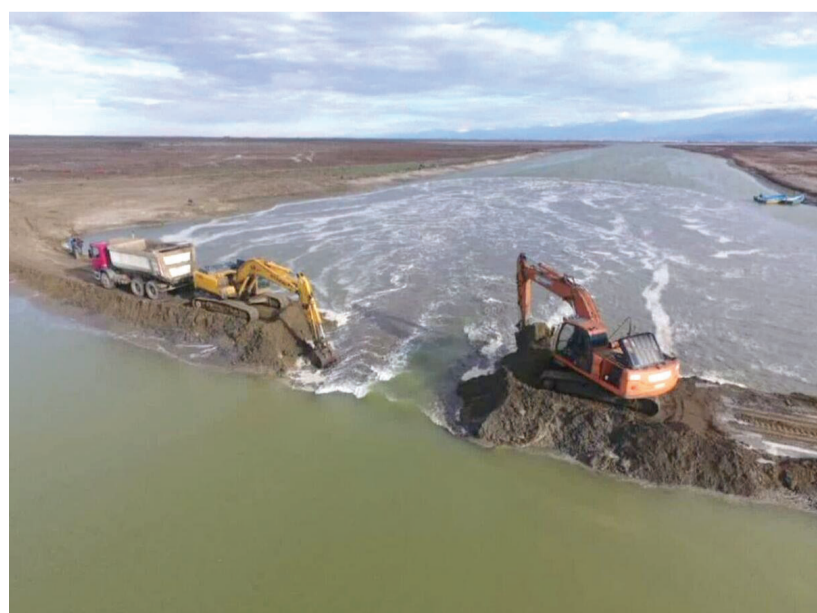
Heavy machinery work to open the Ashuradeh Canal in 2023, allowing water to flow from the Caspian Sea into the drying Gorgan Bay. ● BORNA
