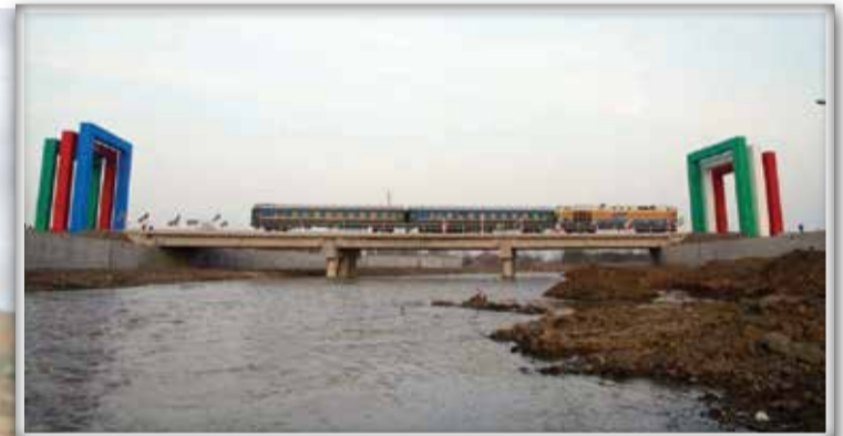
A train crosses a road bridge built between Iran and Azerbaijan over Astarachay.
