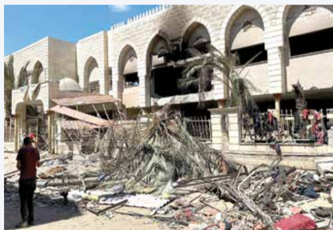
The photo shows the aftermath of an Israeli strike on a school sheltering displaced people in Gaza City on August 10, 2024. ● ABED SABAH/REUTERS
