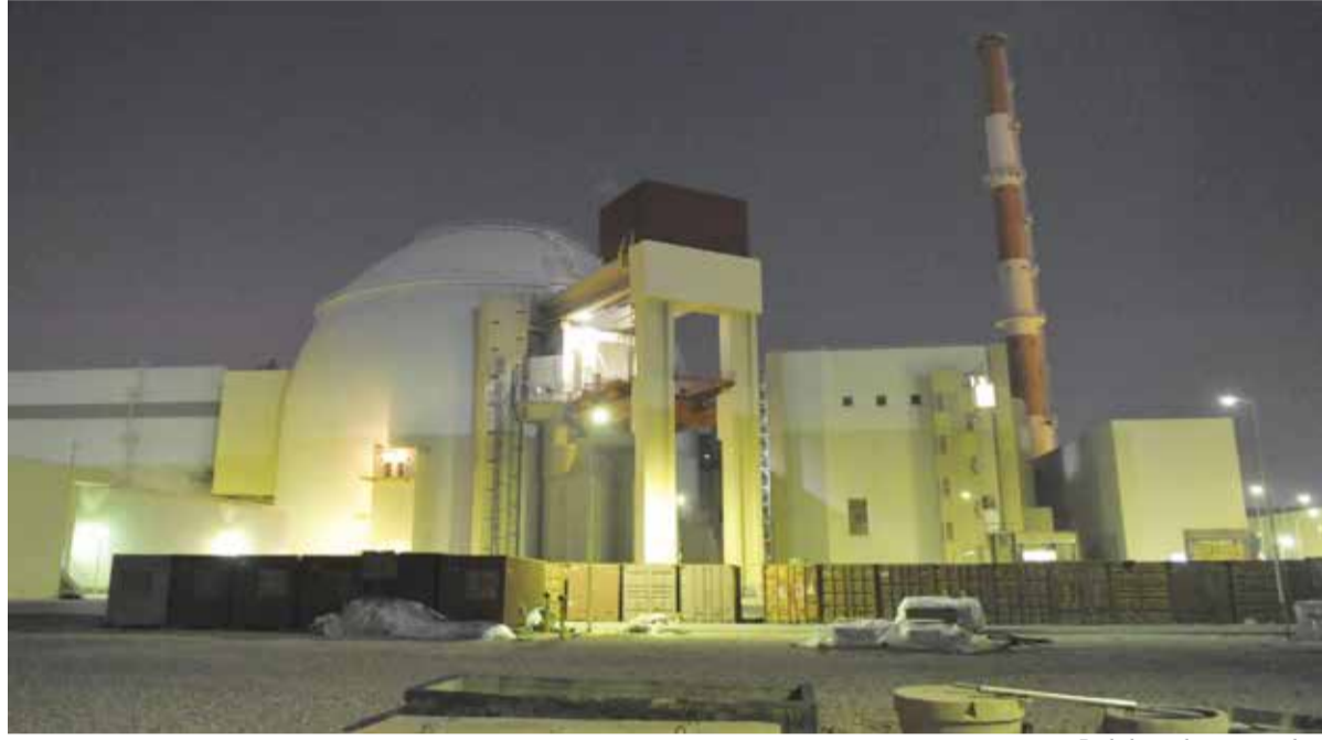
Bushehr nuclear power plant
