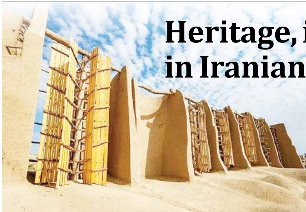
A water mill in Nehbandan ● TASNIM
