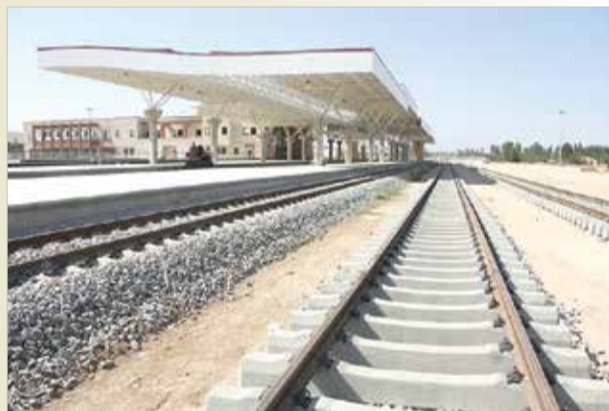
Yazd Railway Station
