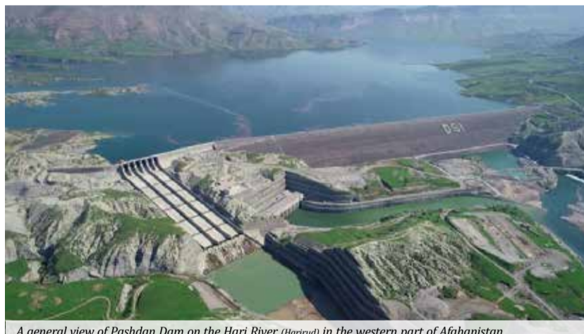
A general view of Pashdan Dam on the Hari River (Harirud) in the western part of Afghanistan
