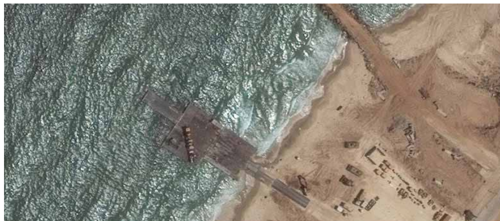
A satellite image on May 29, 2024, shows a view of the remaining section of the dysfunctional pier that was damaged by high winds and heavy seas the week before on the Gaza shoreline. ● MAXAR TECHNOLOGIES/REUTERS
