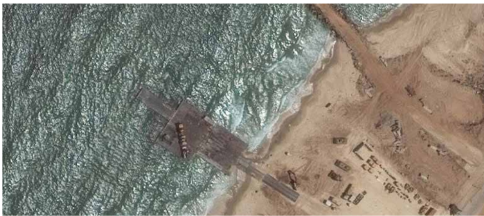
A satellite image on May 29, 2024, shows a view of the remaining section of the dysfunctional pier that was damaged by high winds and heavy seas the week before on the Gaza shoreline. MAXAR TECHNOLOGIES/REUTERS
