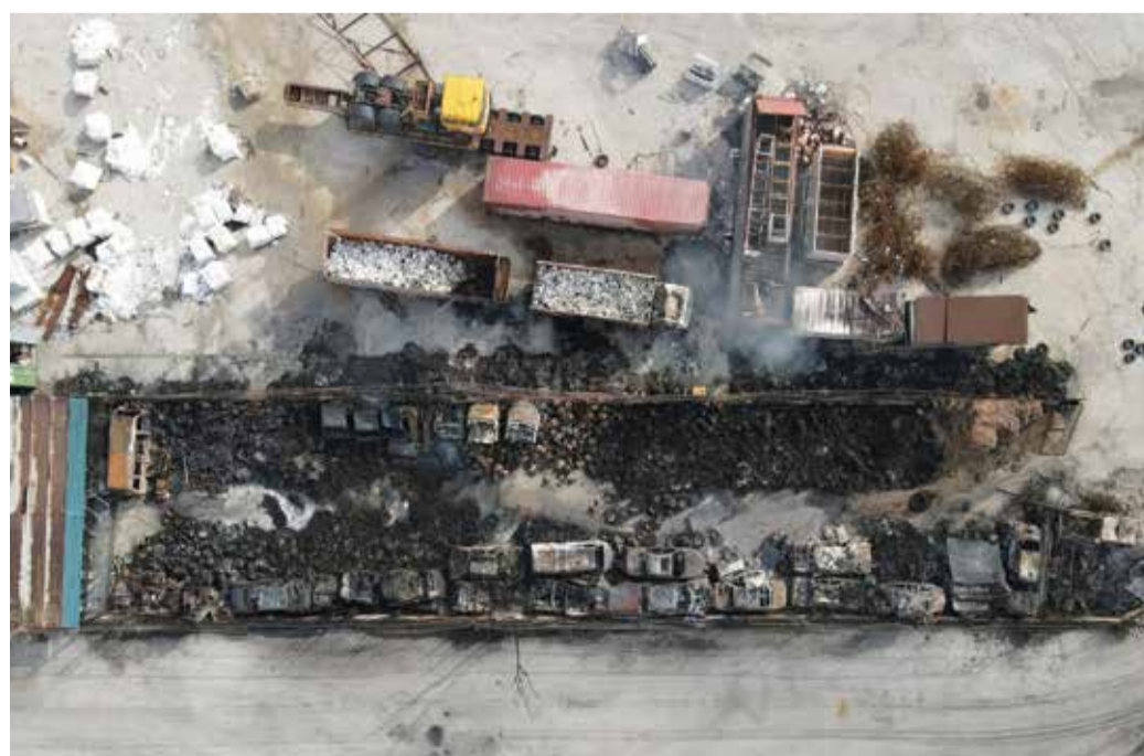
A drone view shows damage at Latakia port after the Israeli military said it struck Syrian defense facilities, Syria, on December 11, 2024.
