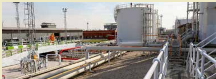
The photo shows Iran's largest oil desalination plant in Ahvaz, southwestern Iran, which was inaugurated remotely by President Masoud Pezeshkian on January 22, 2025.
