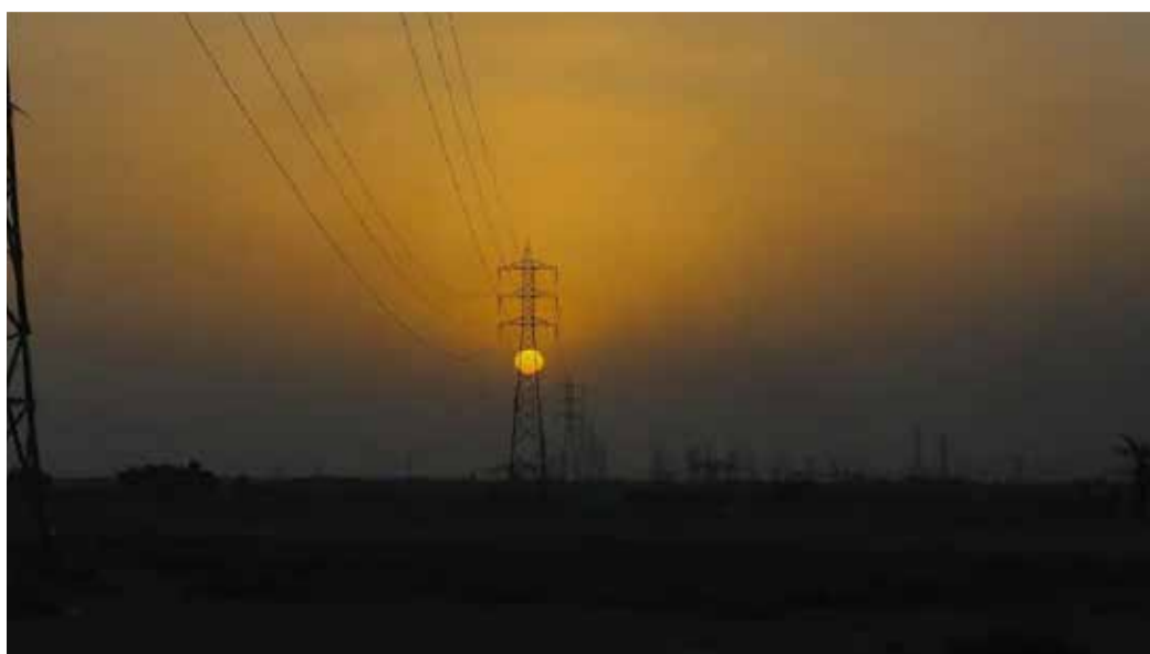
The sun sets behind the transmission lines of electric power from Iran to Iraq in Basra, Iraq, on July 29, 2021. NABIL AL-JURANI/AP
