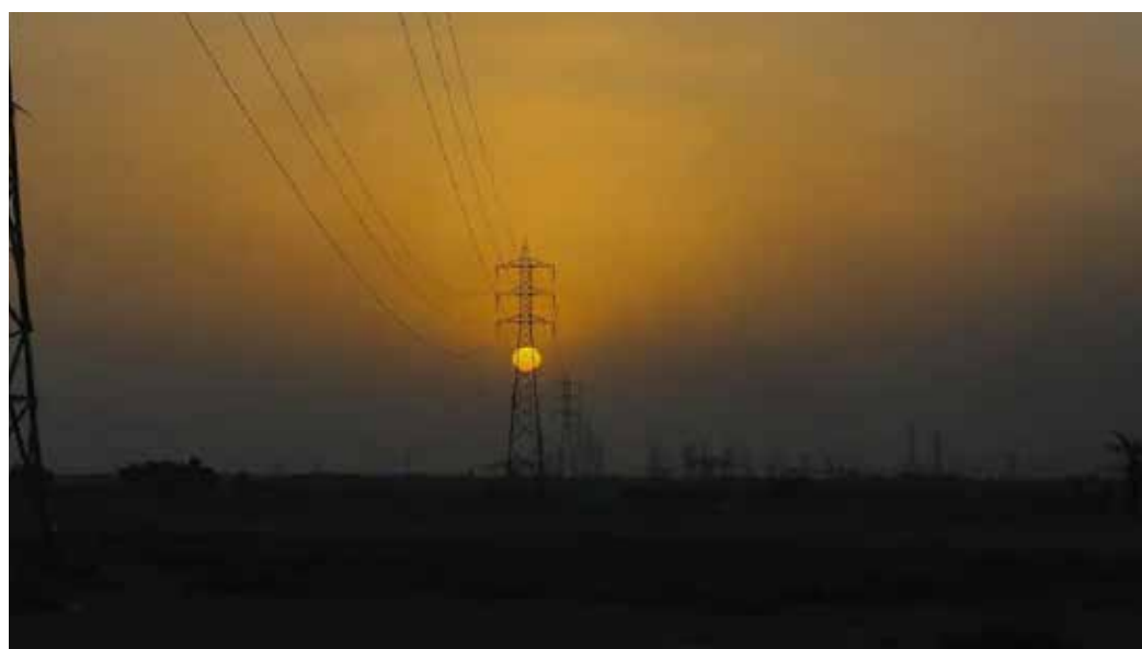
The sun sets behind the transmission lines of electric power from Iran to Iraq in Basra, Iraq, on July 29, 2021.
