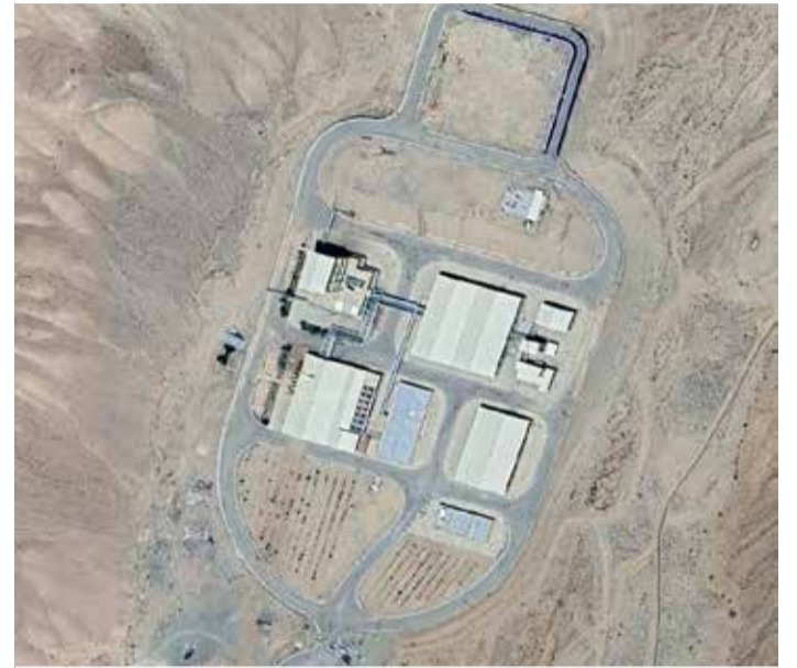
The photo, published by Fox News on May 8, 2025, shows a facility that is claimed to be a secret nuclear site in Iran's Semnan Province.
