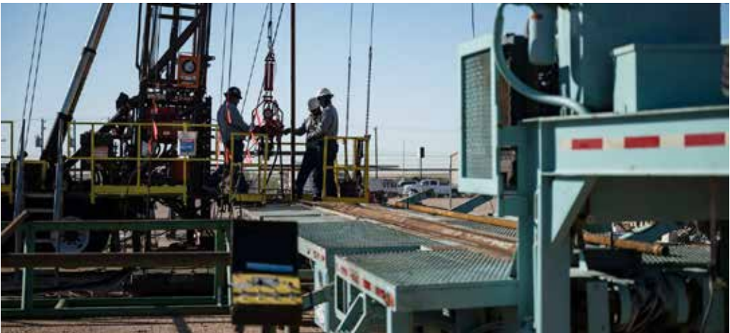
An oilfield crew, contracted by the Railroad Commission of Texas (RRC), works a service rig during a state-funded oil well plugging operation in Midland, Texas, US, on September 25, 2025. ● ELI HARTMAN/BLOOMBERG
