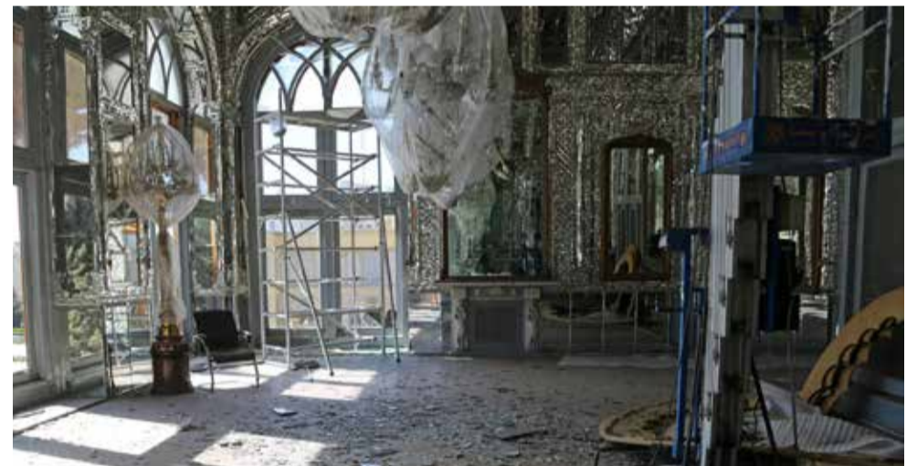
Golestan Palace on March 3, 2026, after it was damaged during US and Israeli airstrikes in Tehran, Iran
