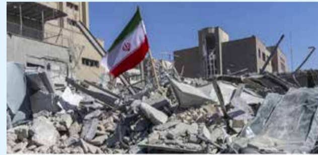
An Iranian flag is planted in the rubble of a police station, damaged in airstrikes on March 3, 2026 in Tehran, Iran. MAJID SAEEDI/GETTY IMAGES
