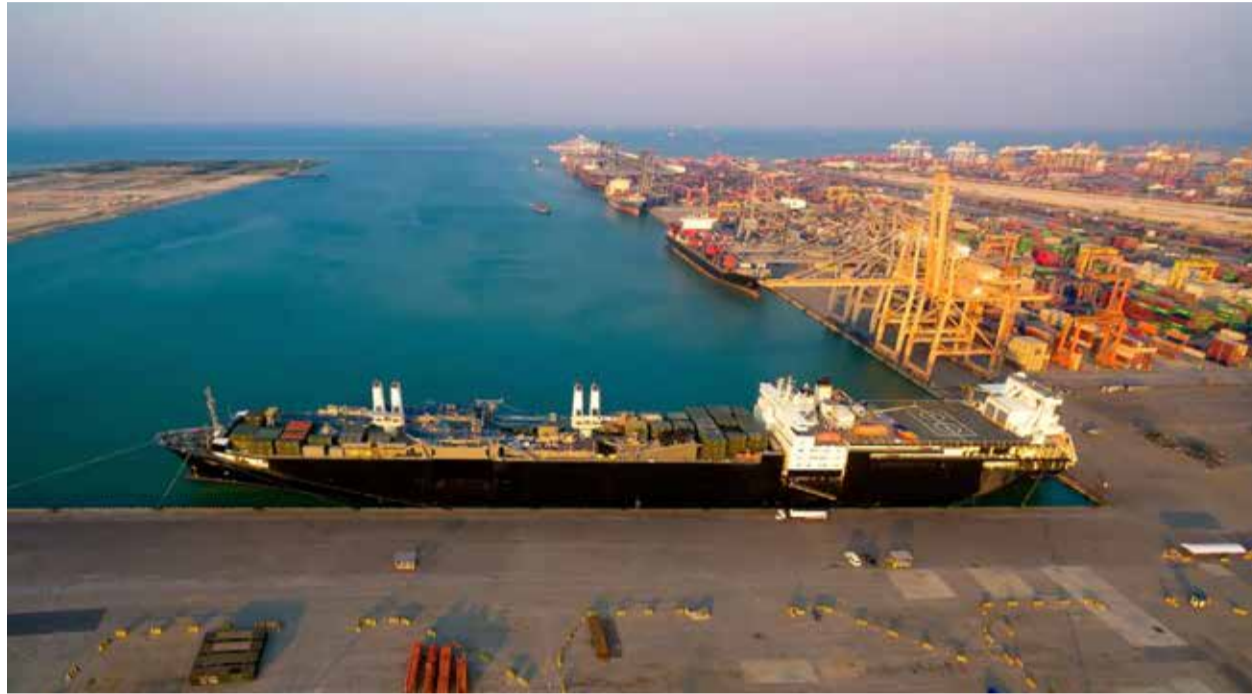
A cargo ship is docked in the Shahid Beheshti terminal in the southeastern Iranian coastal city of Chabahar, on the Gulf of Oman. ● IRNA
