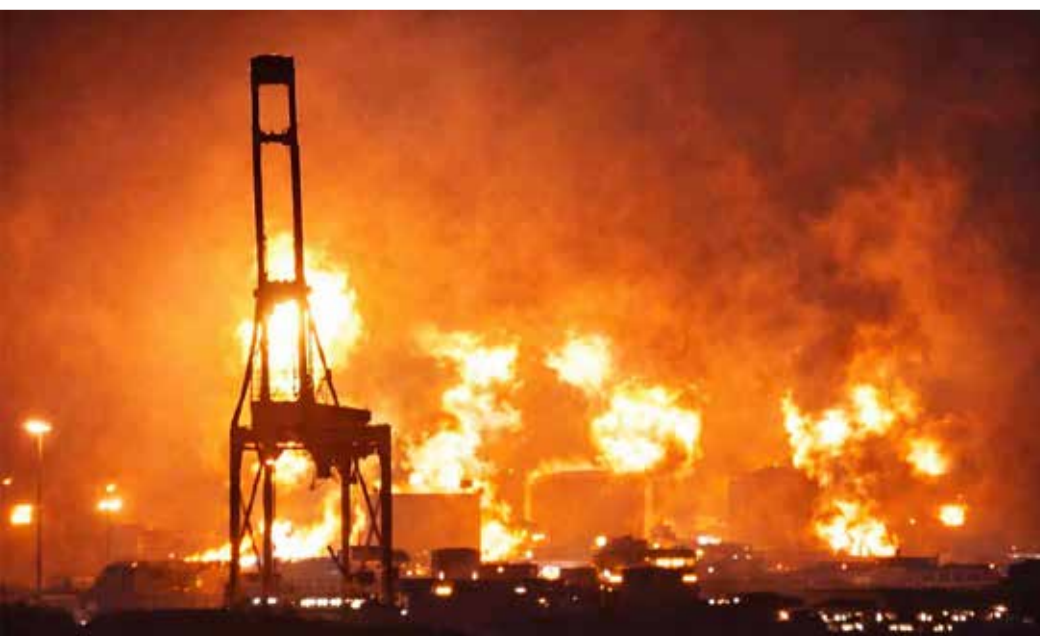
A retaliatory Iranian attack on Qatar's Ras Laffan Industrial City, which houses the world's largest liquefied natural gas (LNG) export facility, has erupted fire and disrupted activities on late March 2026. ● DEFEA PRESS
