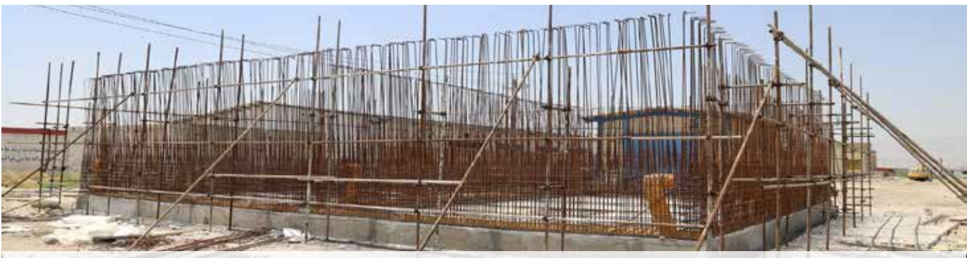
Early construction work for building a desalination plant for the Lamerd Special Economic Zone has been done. ● lamerdsez.ir
