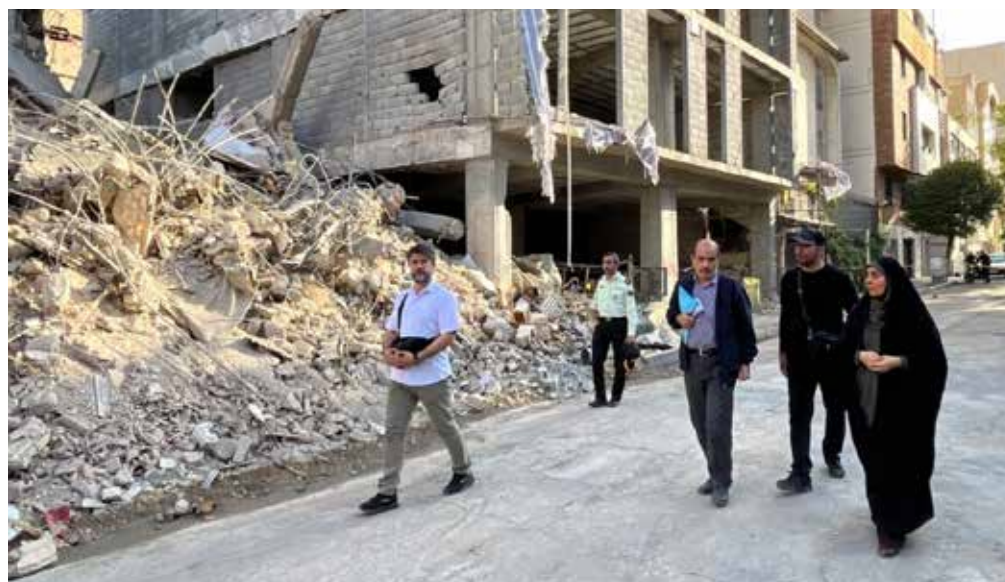
Iran's Minister of Transport and Urban Development Farzaneh Sadegh Malvajerdi (R) visits residential areas damaged in the American-Israeli war in the capital on June 22, 2026. ● IRNA
