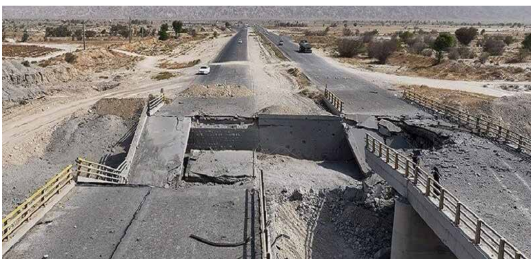
A section of a bridge in Hormozgan Province, southern Iran, has been destroyed on July 17, 2026, after an American missile strike hit this civilian infrastructure. ● IRNA
