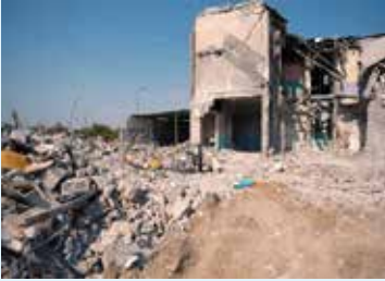
The photo shows the damaged building of the Shajarah Tayyebah Elementary School in the southern Iranian town of Minab, which was targeted by the US military on February 28. ● IRNA
