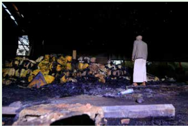
A Yemeni man inspects melted foam inside a factory after a Saudi strike in the Shamlan neighborhood of Yemen's capital Sana'a on October 4, 2026. AFP
