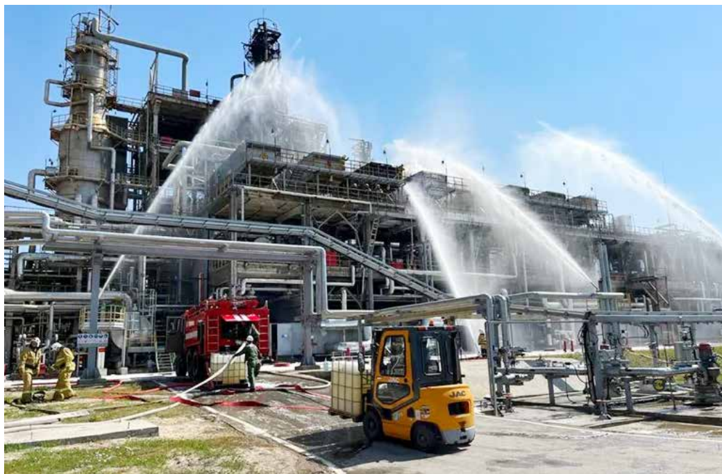
Russian Emergency Situation Ministry's firefighters work at the scene of a fire at the Novoshakhtinsk oil processing plant in the Rostov region on June 22, 2022. ● RUSSIAN EMERGENCY MINISTRY PRESS SERVICE
